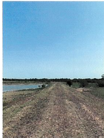
Upstream Flood Control Structure in Rogers County
